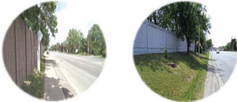
Existing Noise Walls
