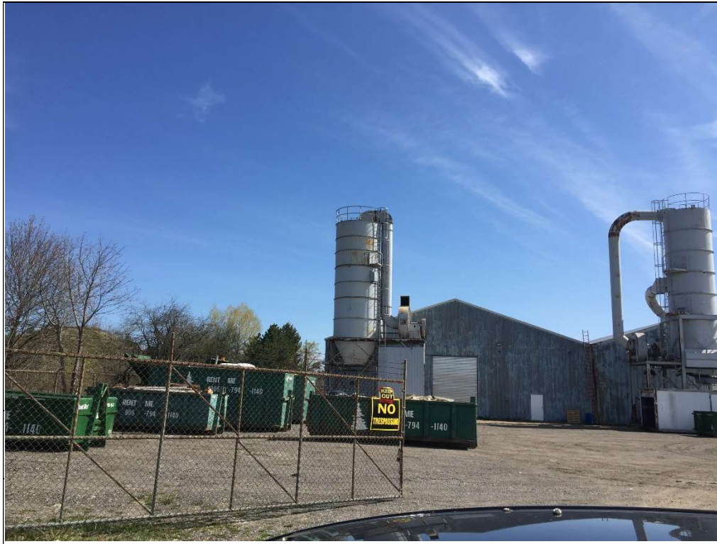
Photo 7: View of the industrial property at 10562 Regional Road 50.
