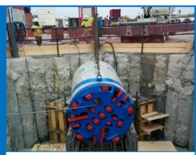
**Microtunnel:** Similar to tunnel, but the machine is smaller and is controlled from the surface.
