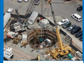
**Tunnel:** Two shafts are dug and the pipe is installed in a tunnel between the shafts.
