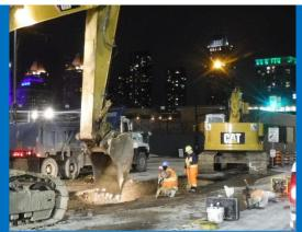
**Open Cut:** A trench is dug, the pipe is installed in the trench and the trench is backfilled.
