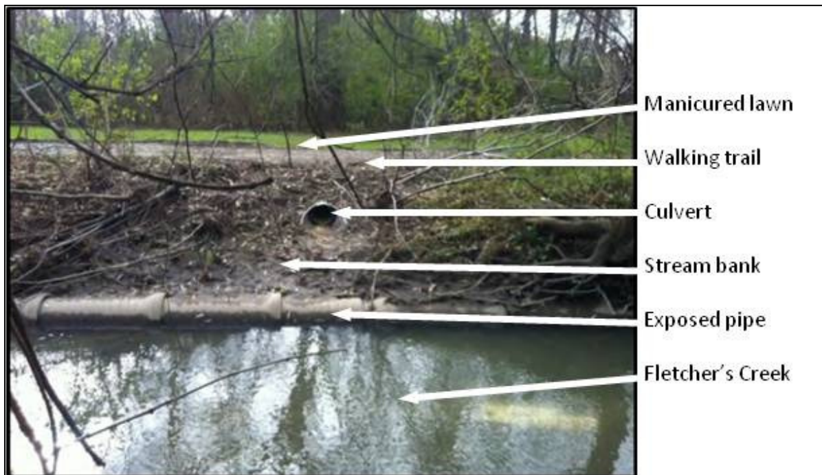
Figure 3- 1: Photograph of exposed pipe in Fletcher's Creek, upstream of Denison Avenue, November, 2012
