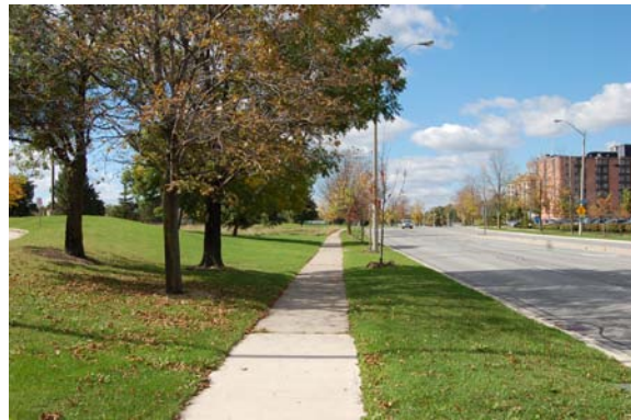
Plate 16: View northwest along Argentia Road. ROW is disturbed. No potential. Lands beyond ROW area graded and disturbed. No potential.
