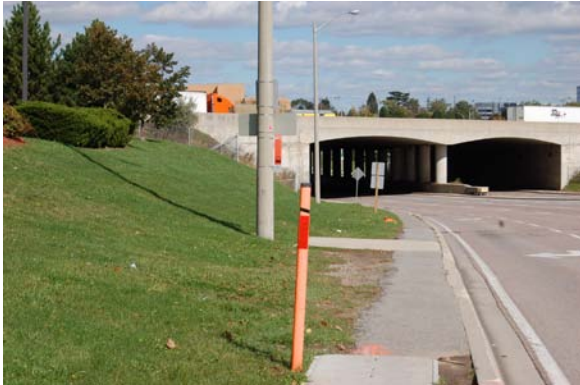
Plate 13: View northeast along Derry Road West. ROW is disturbed. No potential. Lands beyond ROW are also disturbed. No potential.
