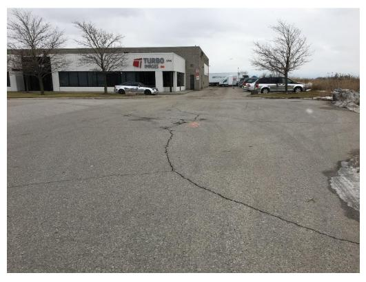
Photo 16: Localized Random Cracking (Moderate Severity)- Menkes Dr
