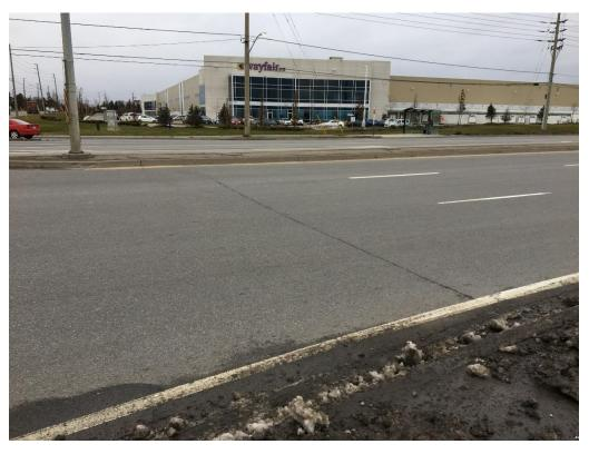
Photo 11: Localized Transverse Cracking (Slight Severity)- Derry Road E NB
