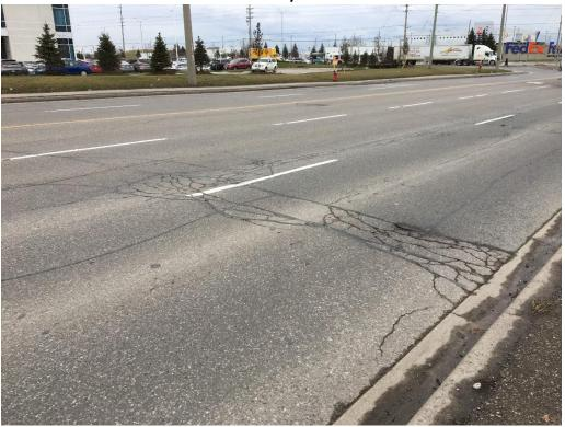
Photo 8: Localized Alligator Cracking (Moderate Severity)-Bramalea Road EB
