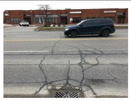
Photo 3: Catch Basin Settlement and Transverse Cracking turning to Alligator Cracking (Slight to Moderate Severity)-Bramalea Road WB
