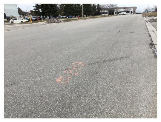
Photo 17: Localized Random Cracking (Slight to Moderate Severity)- Menkes Dr
