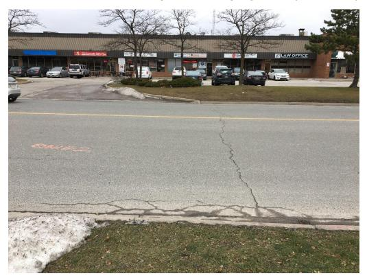
Photo 15: Edge Breaking and Transverse Cracking (Slight to Moderate Severity)- Telford Way
