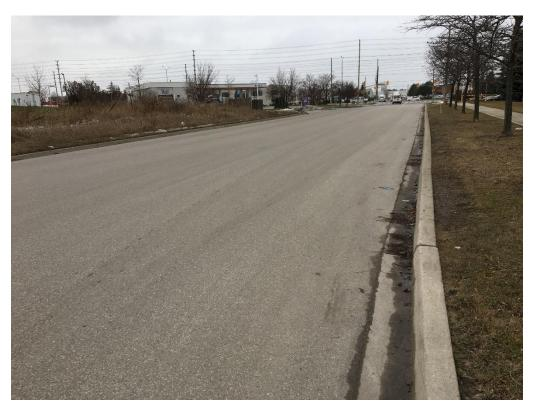
Photo 18: Ravelling (Slight Severity)- Menkes Dr
