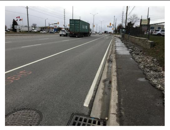
Photo 20: Ravelling (Low Severity)- Derry Road E SB
