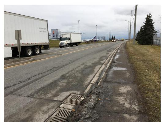
Photo 9: Transverse and Longitudinal Cracking (Slight to Moderate Severity)-Bramalea Road EB
