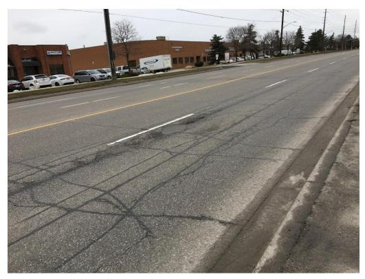
Photo 4: Localized Potholes and Cracking (Slight to Moderate Severity)-Bramalea Road WB
