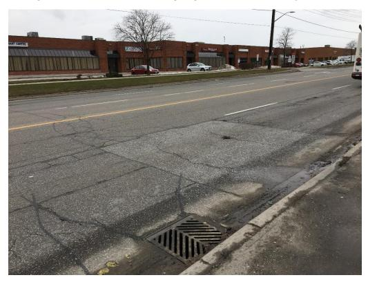
Photo 2: Localized Patch and Alligator Cracking (Slight to Moderate Severity)- Bramalea Road WB
