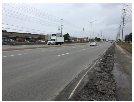
Photo 19: Ravelling (Slight Severity)- Derry Road E NB
