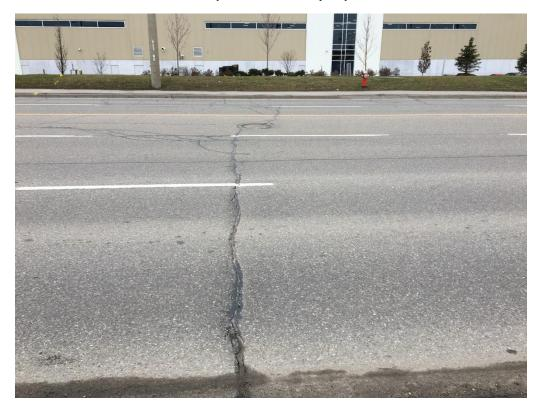
Photo 6: Transverse Cracking (Moderate Severity)-Bramalea Road EB
