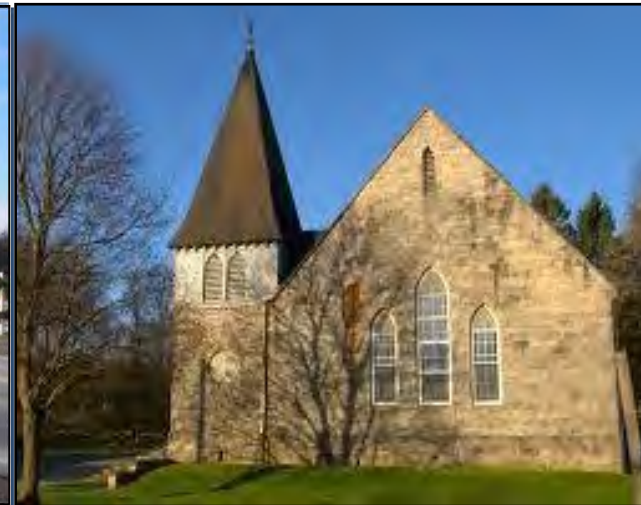
Belfountain Village Church
