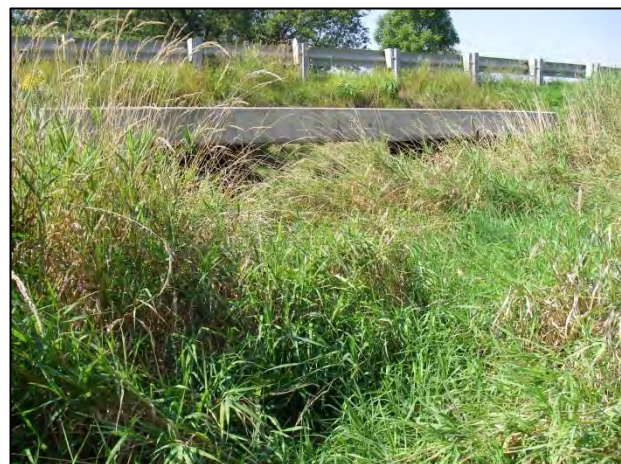
Downstream end of culvert facing upstream (west)
