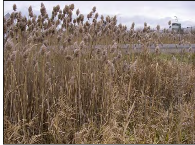
Upstream end of culvert facing downstream (east)
