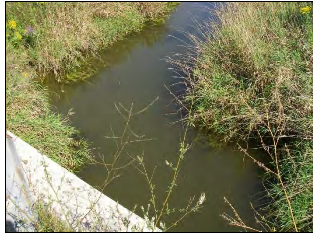
Pool/ponded area upstream of culvert
