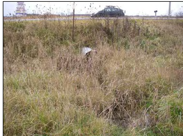
Downstream end of culvert facing upstream (west)
