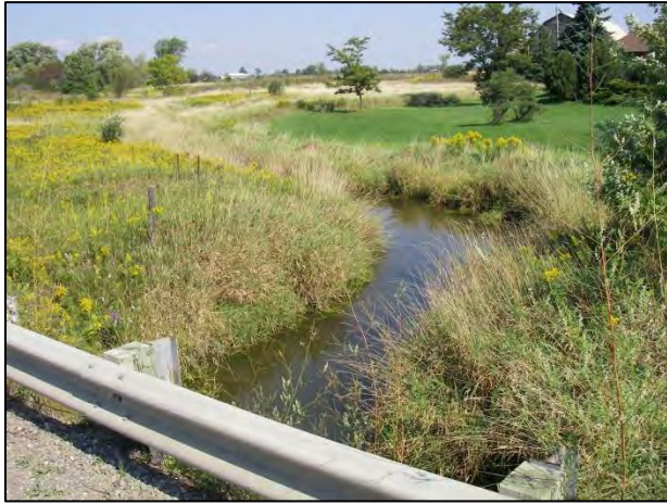
Salt Creek upstream (east) of culvert. Note ponding
