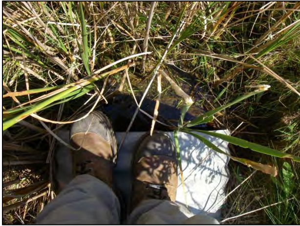
Upstream (east) end of culvert showing small amount of standing water within cattails
