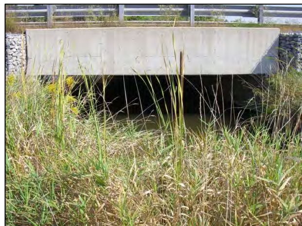
Downstream end of culvert facing upstream (east)
