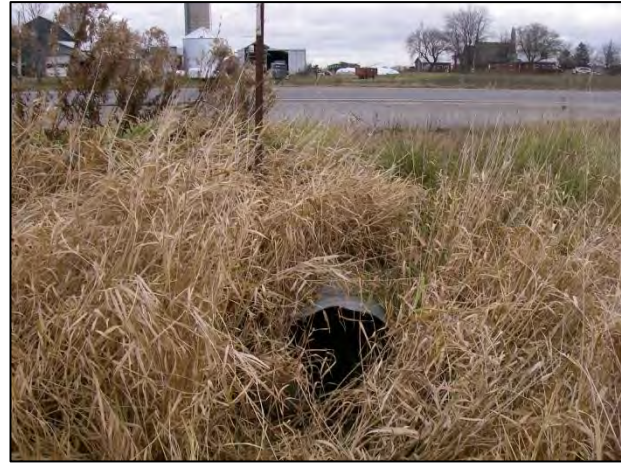
Upstream end of culvert facing downstream (east)
