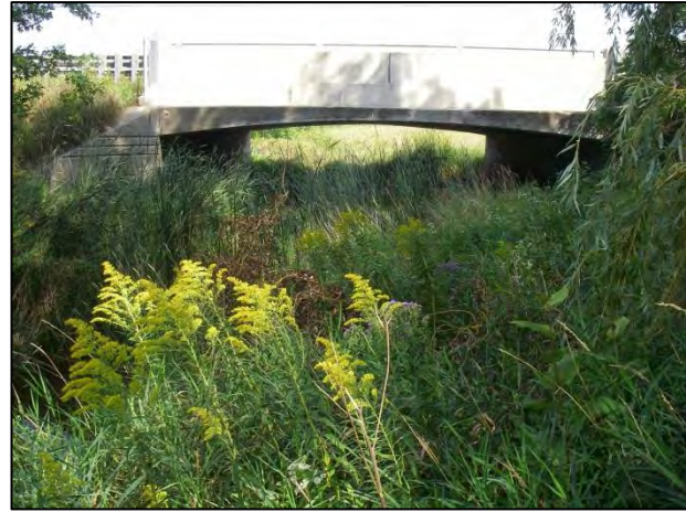
Upstream end of bridge facing downstream (east)
