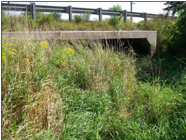
Facing downstream (east) at upstream end of culvert
