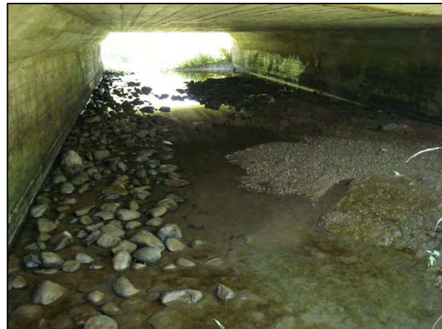
Inside culvert. Photo taken from downstream end facing upstream
