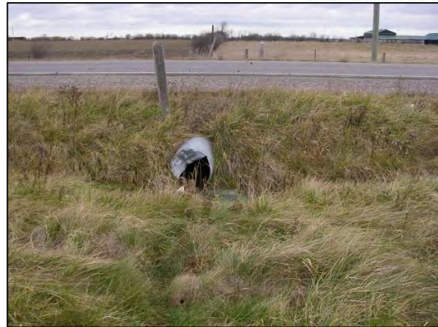
Upstream end of culvert facing downstream (east)
