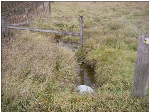
Facing downstream (east) at downstream end of culvert
