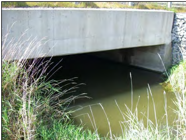
Upstream (east) end of culvert facing downstream
