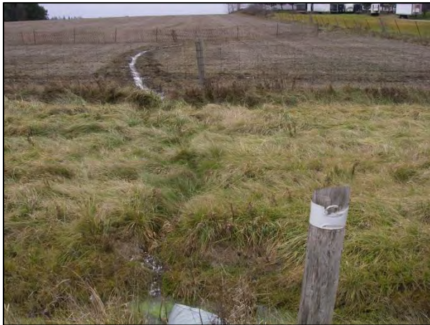
Tributary of Salt Creek facing upstream (west) from upstream end of culvert
