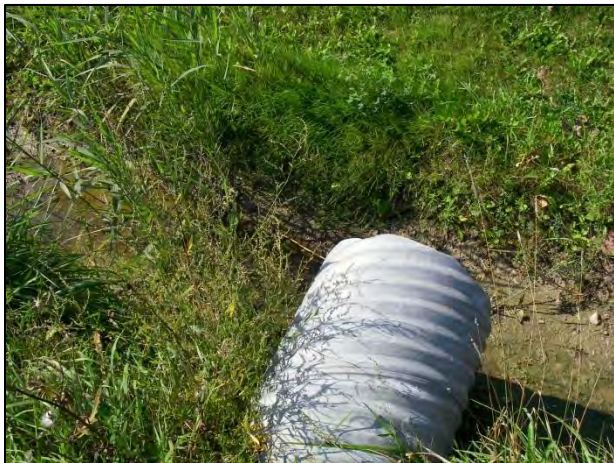
Downstream (west) end of culvert
