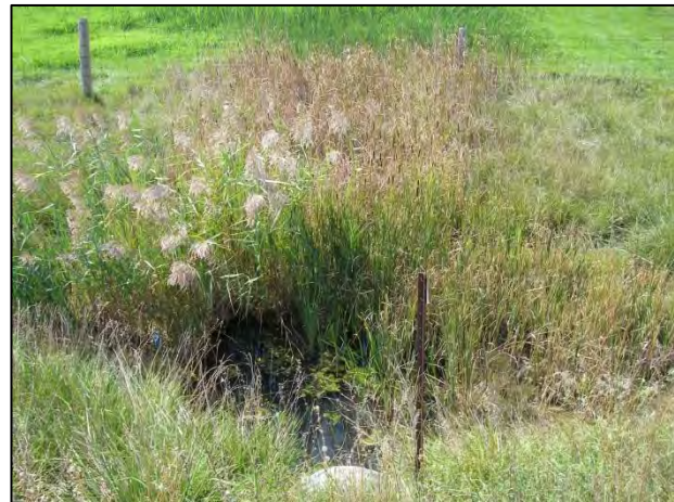
Downstream (west) end of culvert facing downstream
