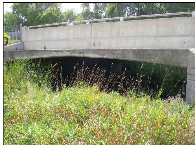
Downstream end of bridge facing upstream (west)
