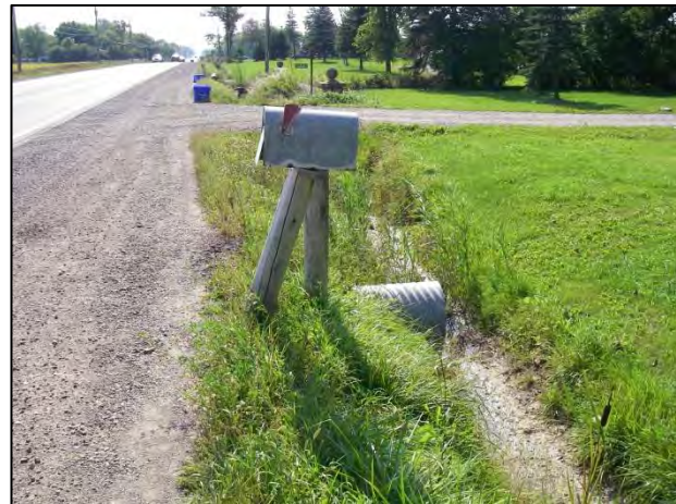
Downstream end of culvert facing south
