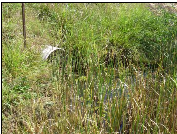
Downstream end of culvert showing small amount of standing water
