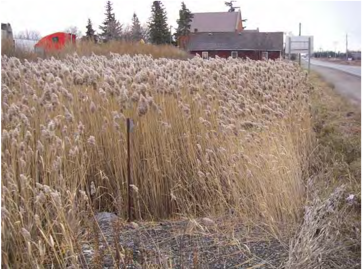
Culvert 11 (TRCA Crossing ID 8) Downstream End
