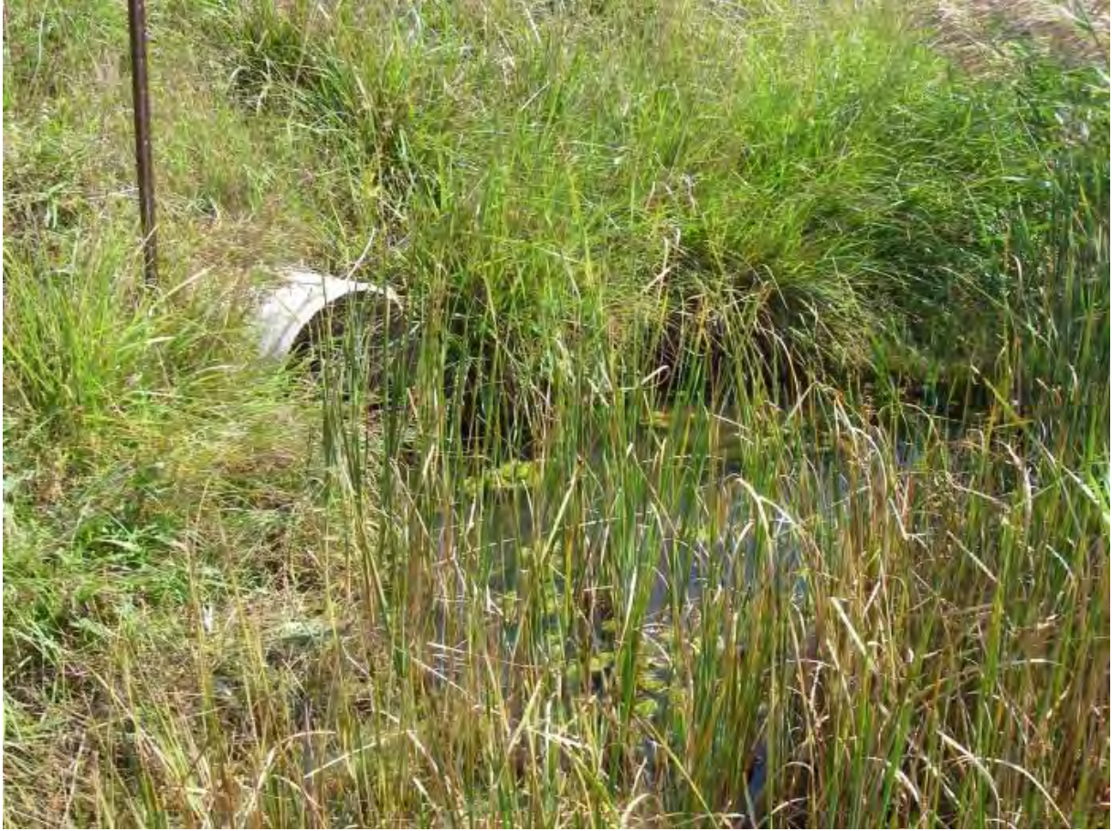
Culvert 4 (C4 -TRCA Crossing 3) Downstream End
