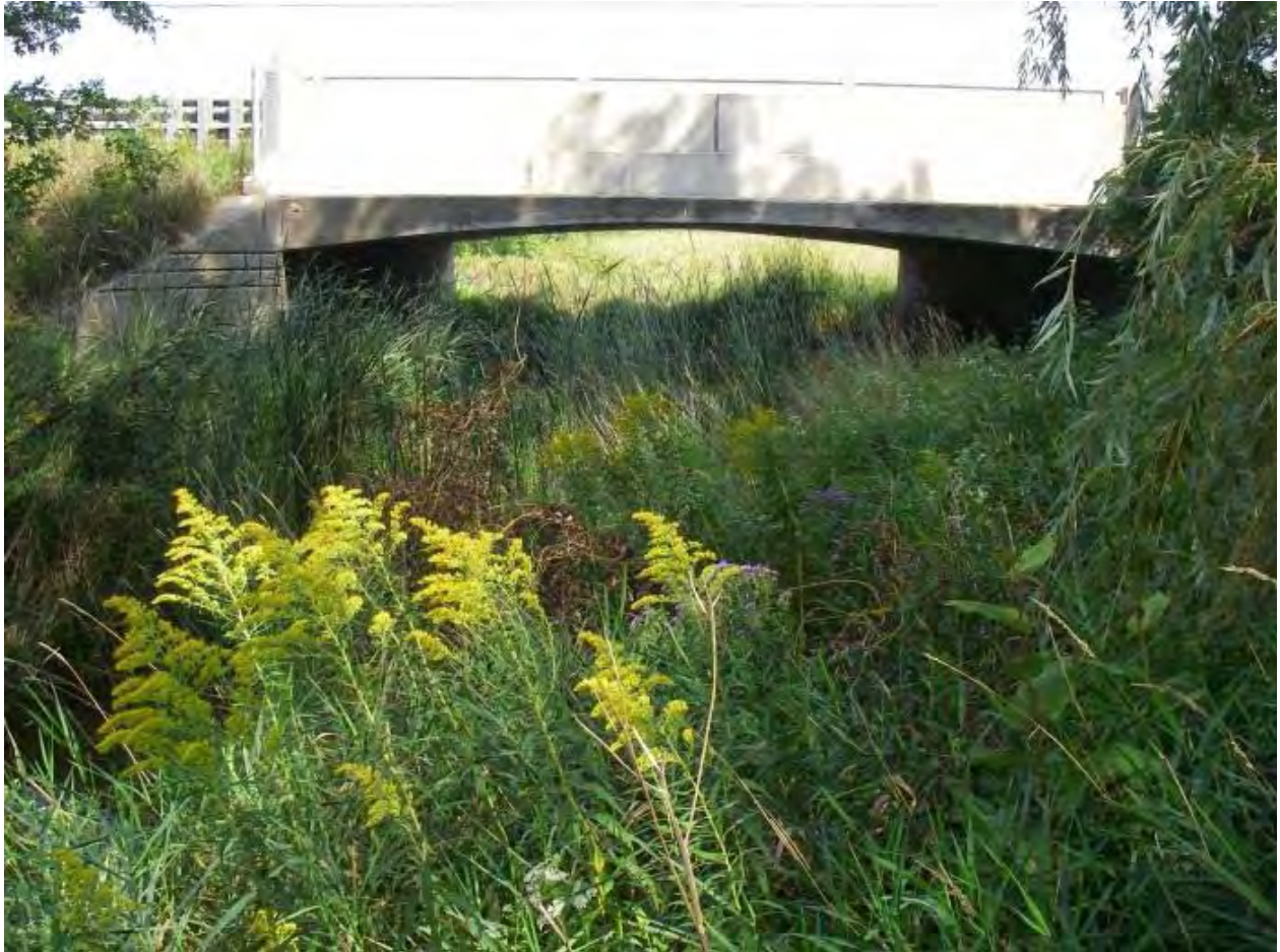
Norris Bridge (C2 -TRCA Crossing ID 2) Upstream End
