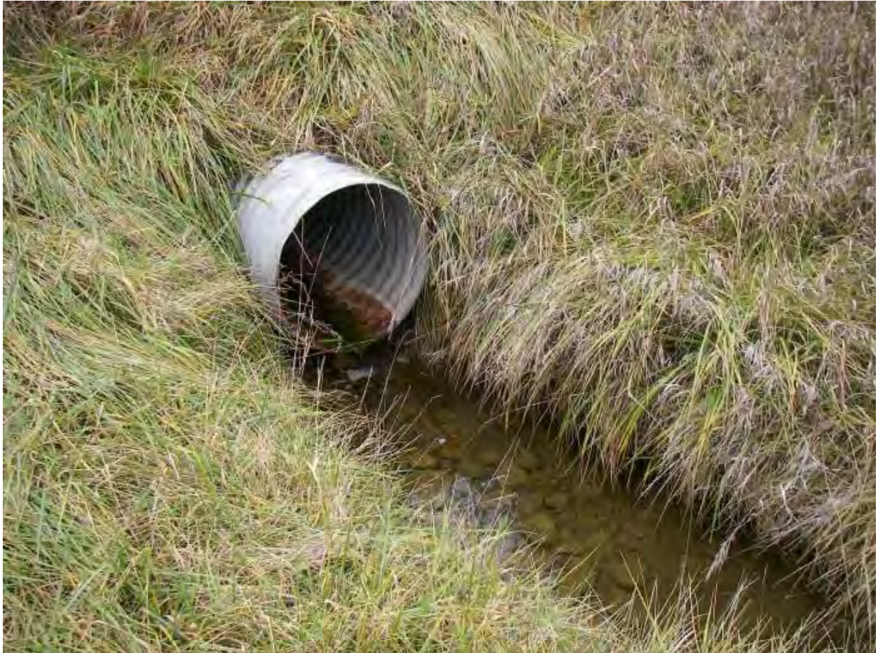
Culvert 10 (TRCA Crossing ID 7) Downstream End
