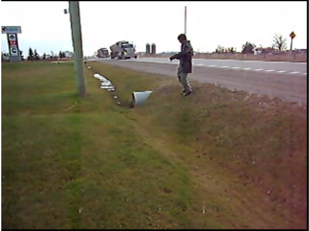
Culvert 5 (Approximately 250m North of Old School Road) Upstream End
