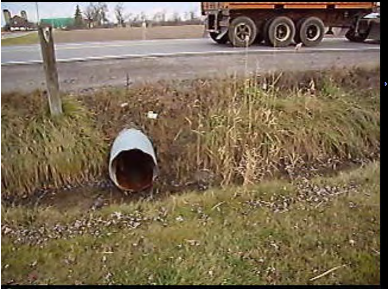
Culvert 8 (TRCA Crossing ID 6) Downstream End
