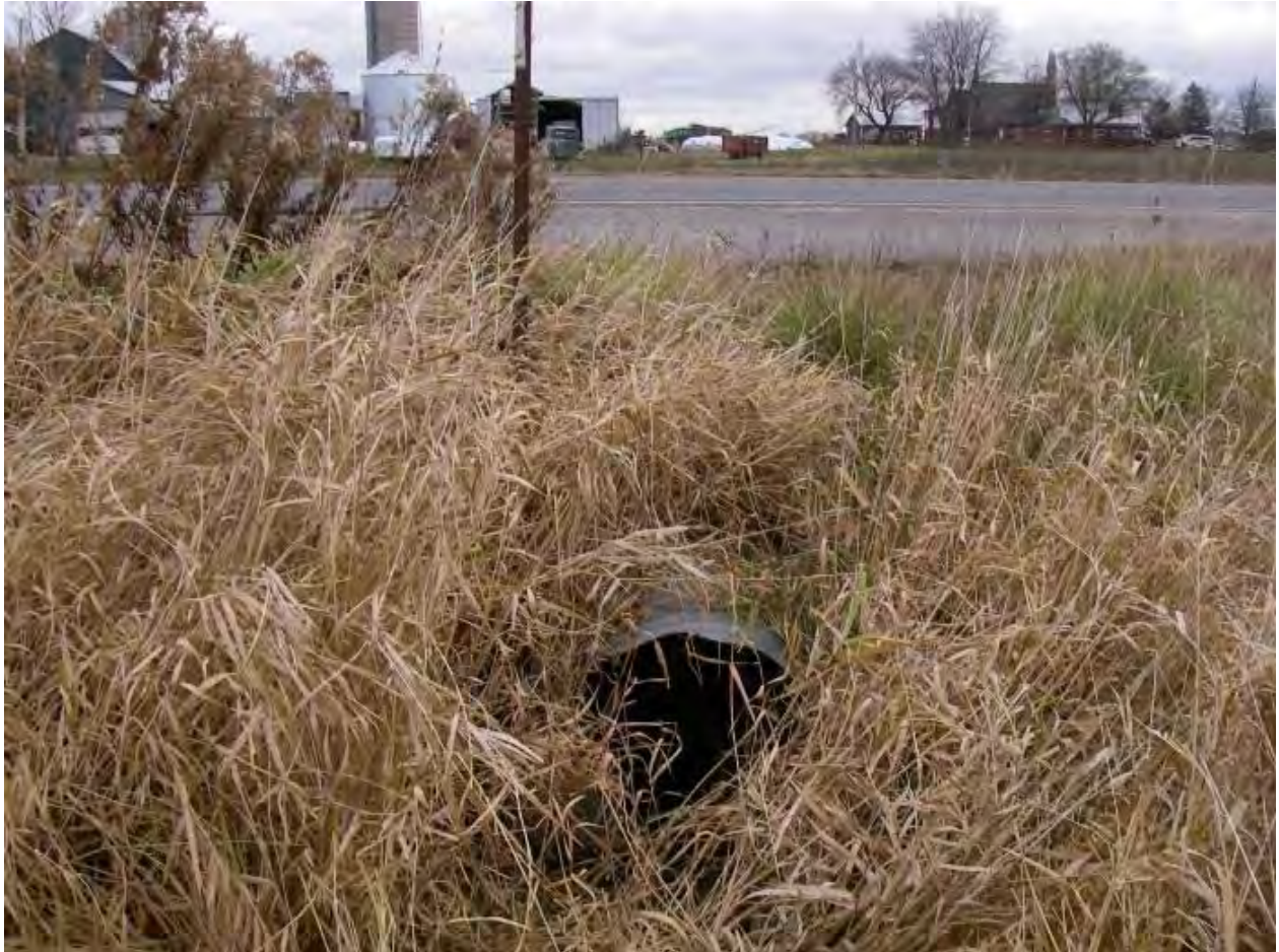
Culvert 13 (TRCA Crossing ID 9 Upstream End)
