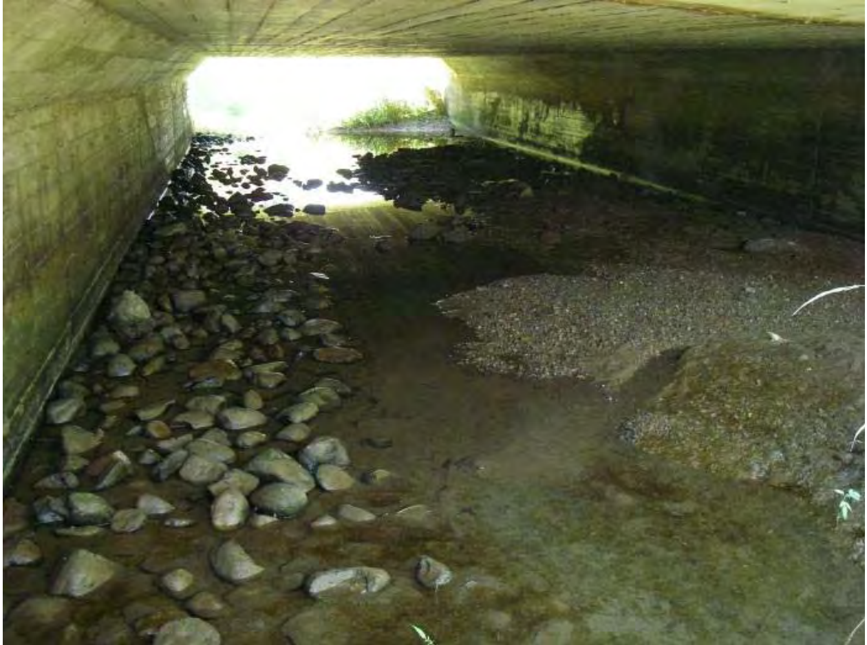
Salt Creek Culvert (C7- TRCA Crossing ID 5)
