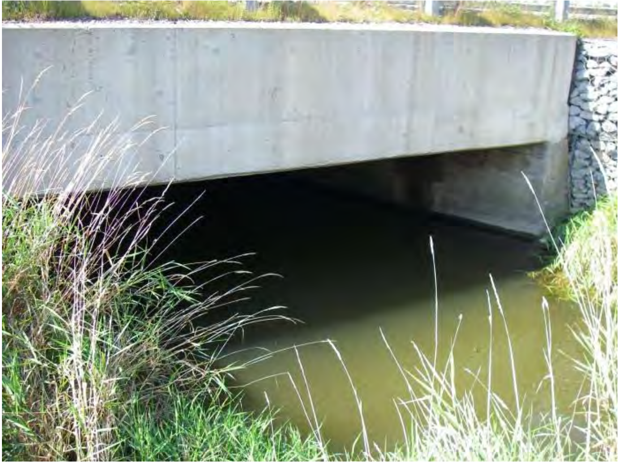
Deans Culvert (C6-TRCA Crossing ID 4) Upstream End
