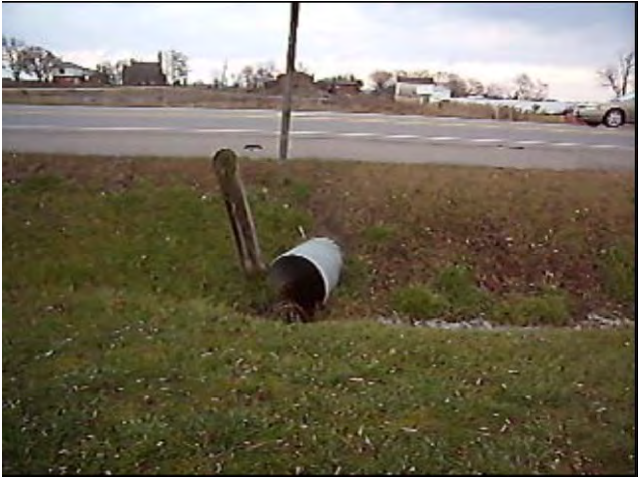
Culvert 12 (Approximately 50m South of King Street) Upstream End
