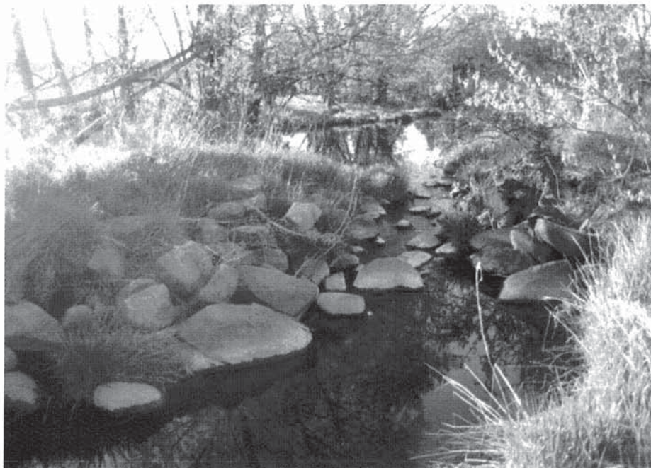
Photo 4. Channel narrowing and rip-rapped banks at old farm crossing
