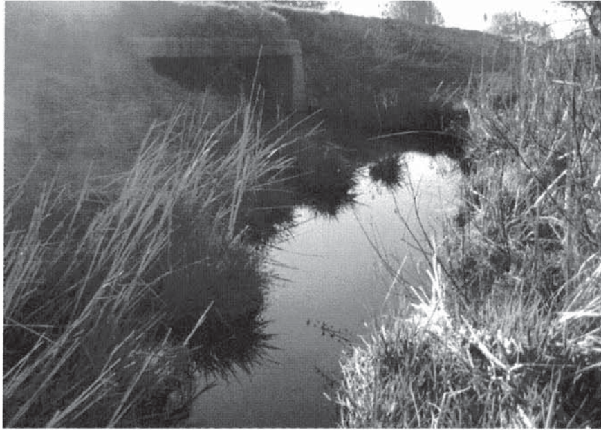
Photo 7. Inlet of existing culvert (C3) beneath Mississauga Road
