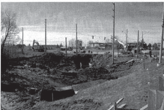
Plate 5: View along illustrating disturbance where additional sewer shafts are being installed.
