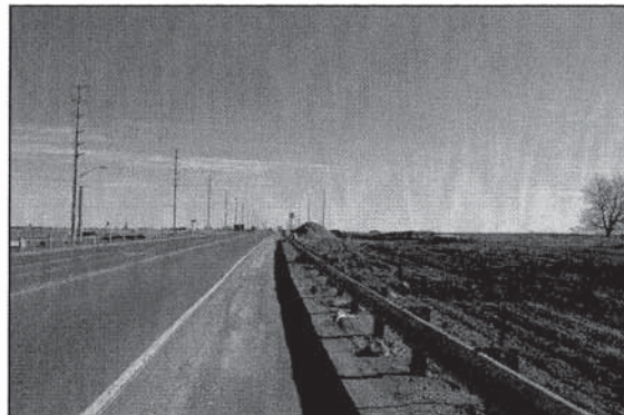
Plate 2: View northeast along south side of Bovaird Street.
