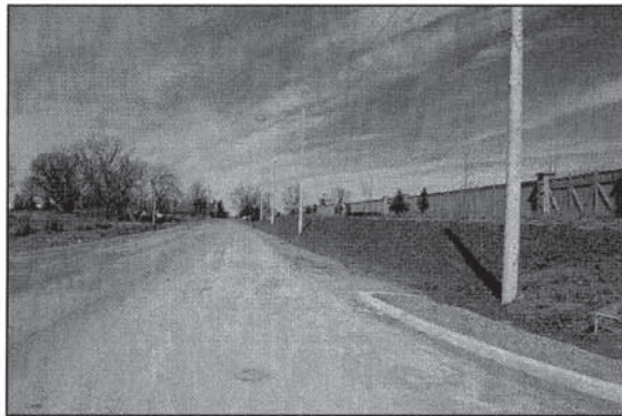
Plate 28: View northwest along Creditview Road (east side).
