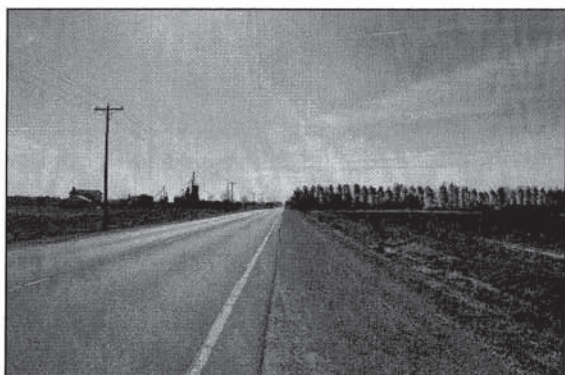
Plate 9: View southeast along Mississauga Road (west side).
