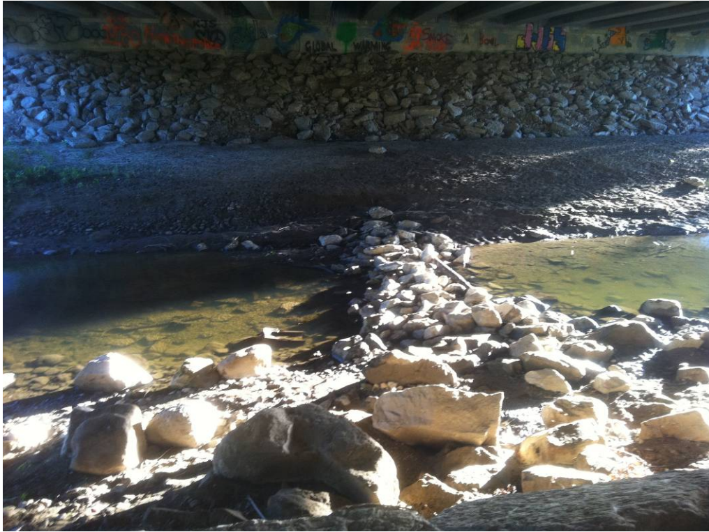
Photo 3: Barrier beneath Snelgrove Bridge. View looking east. Photo was taken September 4, 2011.
