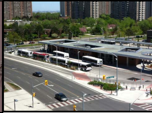
Transit Bramalea City Centre Bus Terminal
