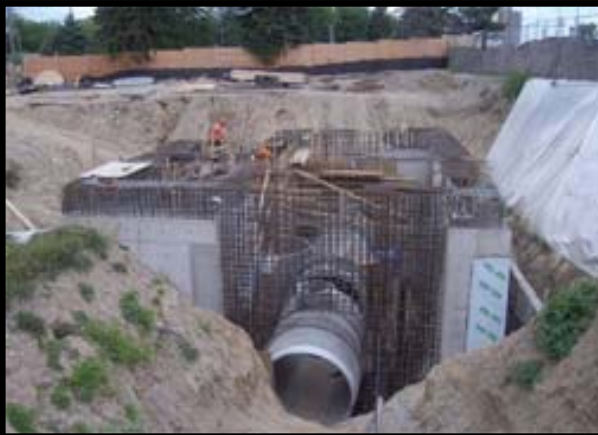
Optimize Community Infrastructure Hanlan Water Project
