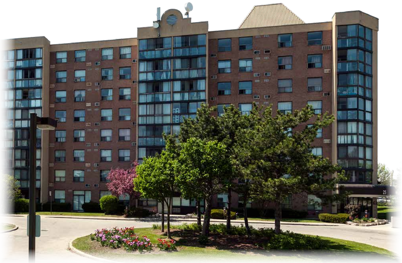
The Region of Peel's affordable housing community on Glenn Hawthorne Blvd., Mississauga
