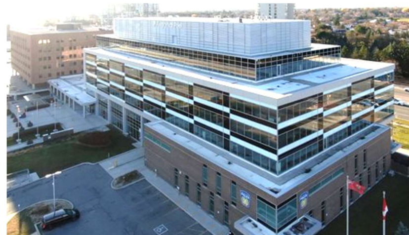
Region of Peel Headquarters at 10 Peel Centre Drive
