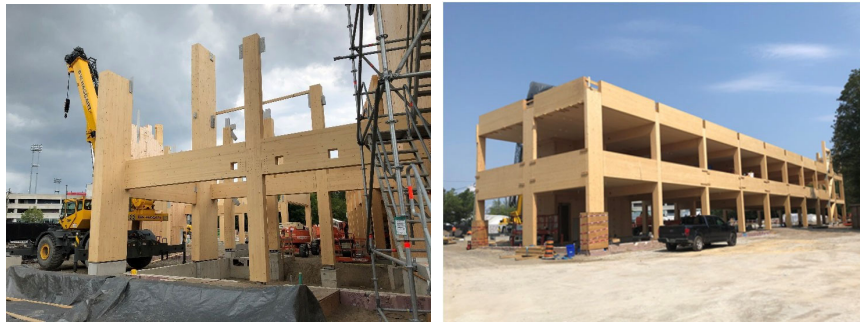
TRCA's New Administrative Office Building
