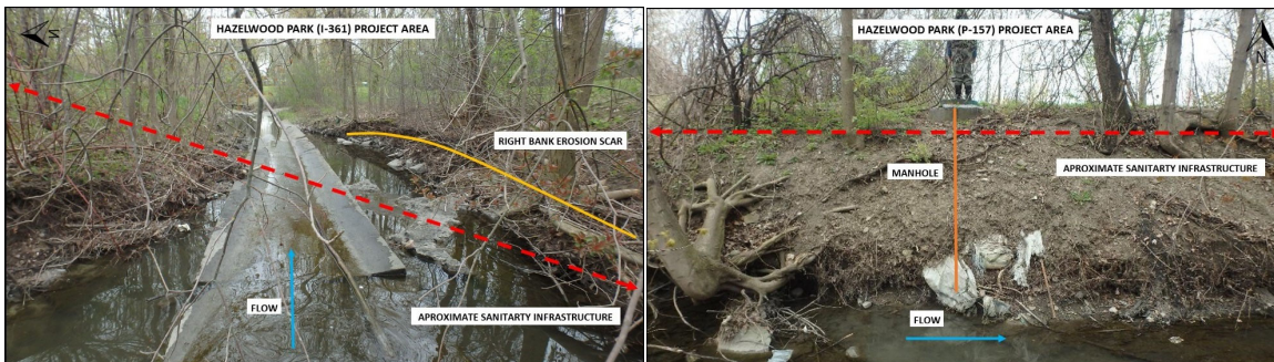
Two of the Hazelwood Park Sanitary Infrastructure Protection Project Sites, planning & design phase
