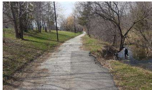
Brandon Gate Park Bank Stabilization Project Site
